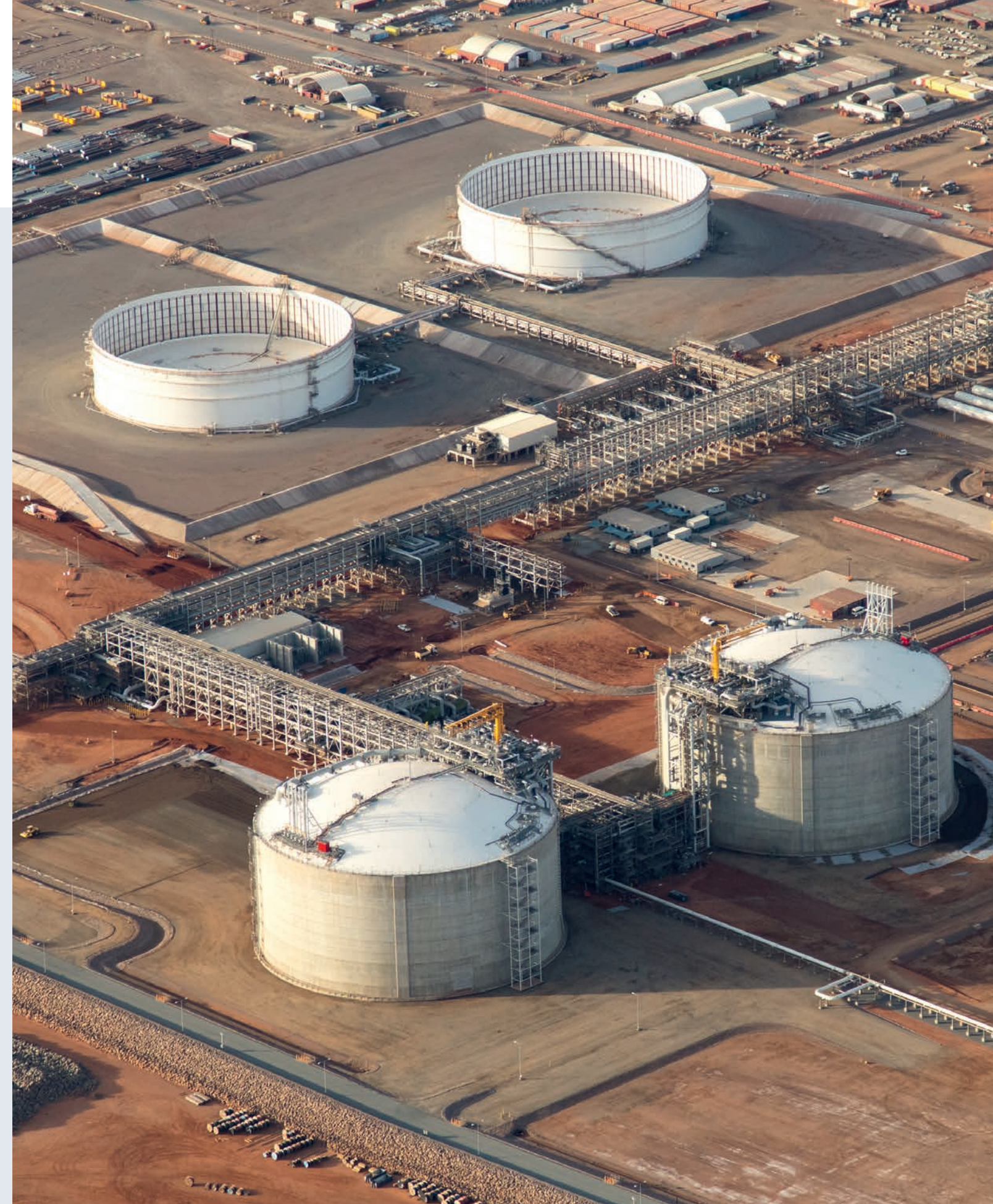
The Wheatstone project's two full containment LNG tanks and two condensate tanks, Australia
