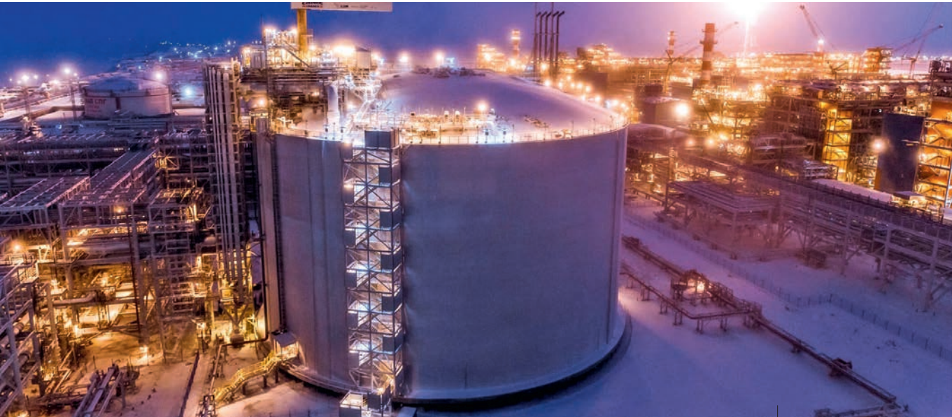
Full containment cryogenic tanks at Yamal LNG, Russia
