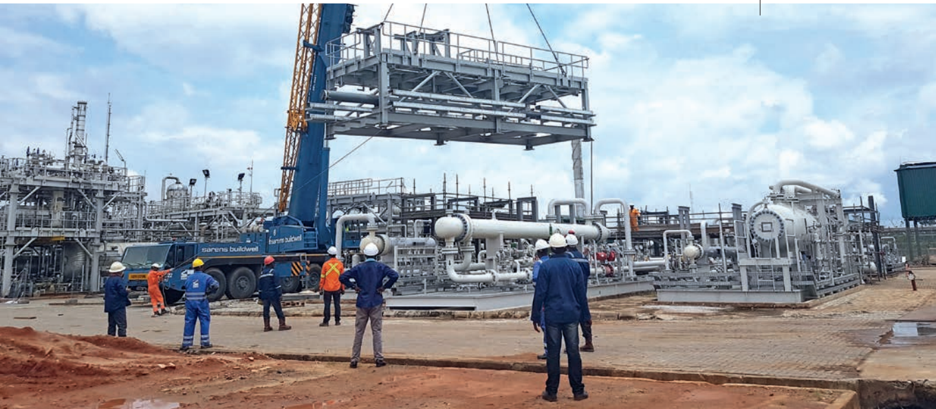
Heavy lifting operation at Oben gas processing plant, Nigeria
